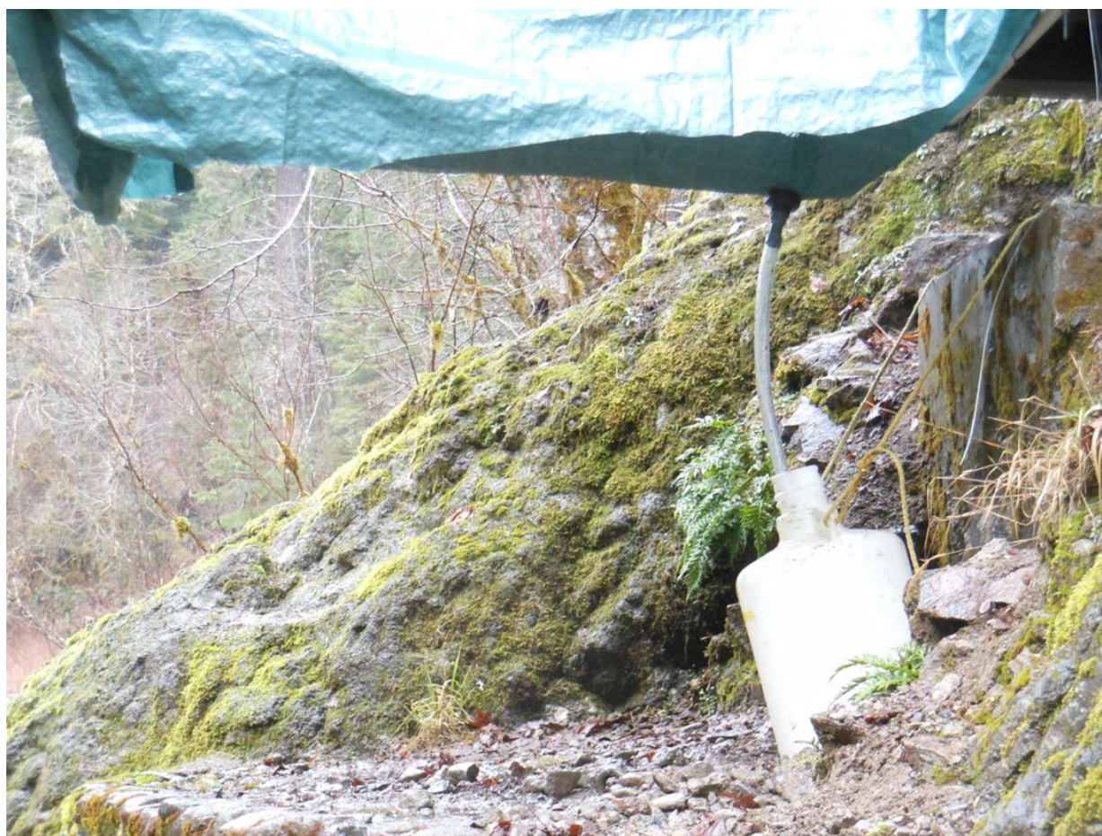
Figure 15. System used to collect water from the House Rock Bridge located near Upper Soda, Oregon.
