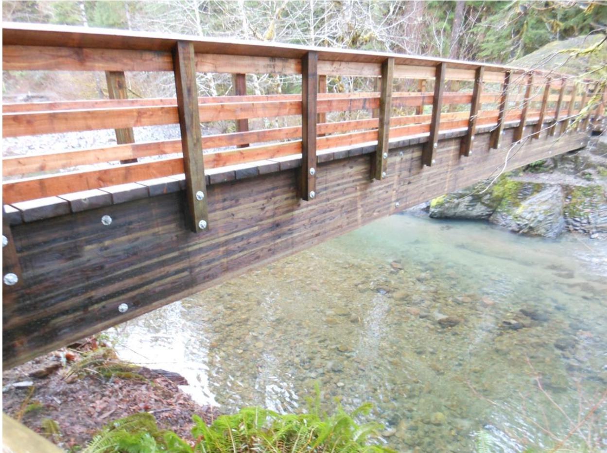
Figure 14. Photograph of the House Rock Bridge showing copper naphthenate treated laminated beams and pentachlorophenol treated decking.
