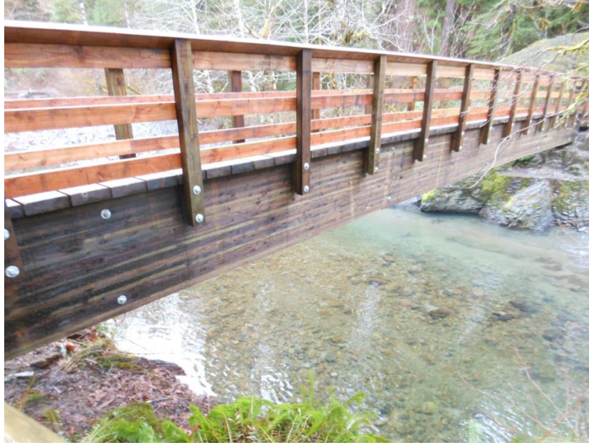
Figure 2. Photograph of the House Rock Bridge showing copper naphthenate treated laminated beams and pentachlorophenol treated decking.
