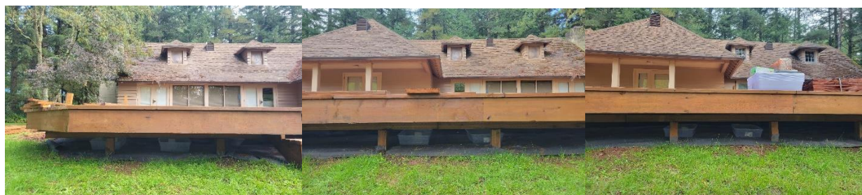
Figure 1.5.1: Placement of water collection basins under the all-new portion of the Peavy Lodge deck at collection site 1 (left), site 2 (middle) and site 3 (right).
