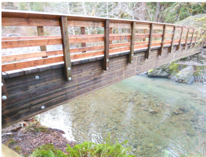
Figure 22. Photograph of the House Rock Bridge showing copper naphthenate treated laminated beams and pentachlorophenol treated decking.
