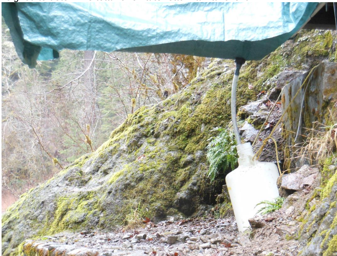
Figure 23. System used to collect water from the House Rock Bridge located near Upper Soda, Oregon.
