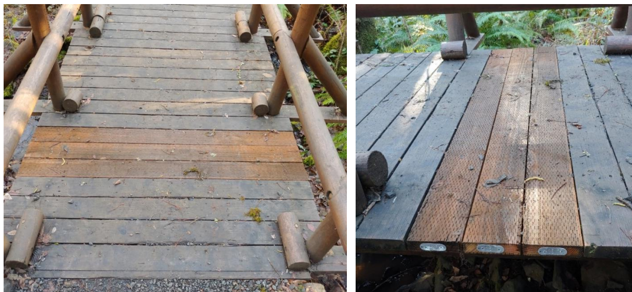
Figure 1.3.1. Deck boards used to assess abrasion rates in the bridge at Peavy Arboretum.
