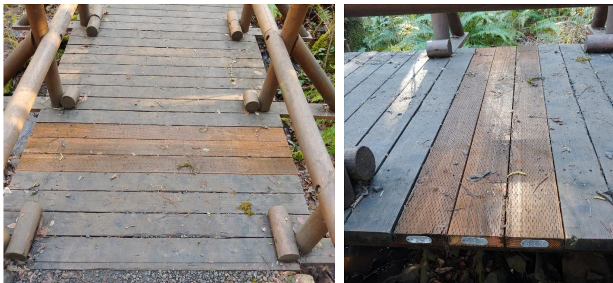
Figure 7. Deck boards used to assess abrasion rates in the bridge at Peavy Arboretum.
